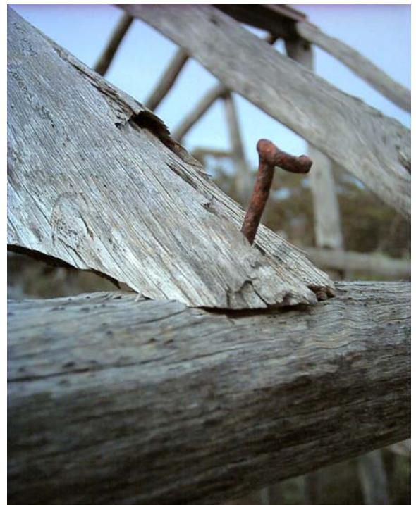
Close-up of fencing wire used as a nail at Burnabbie ruins. Peter Ackroyd, 17 April 2007.
